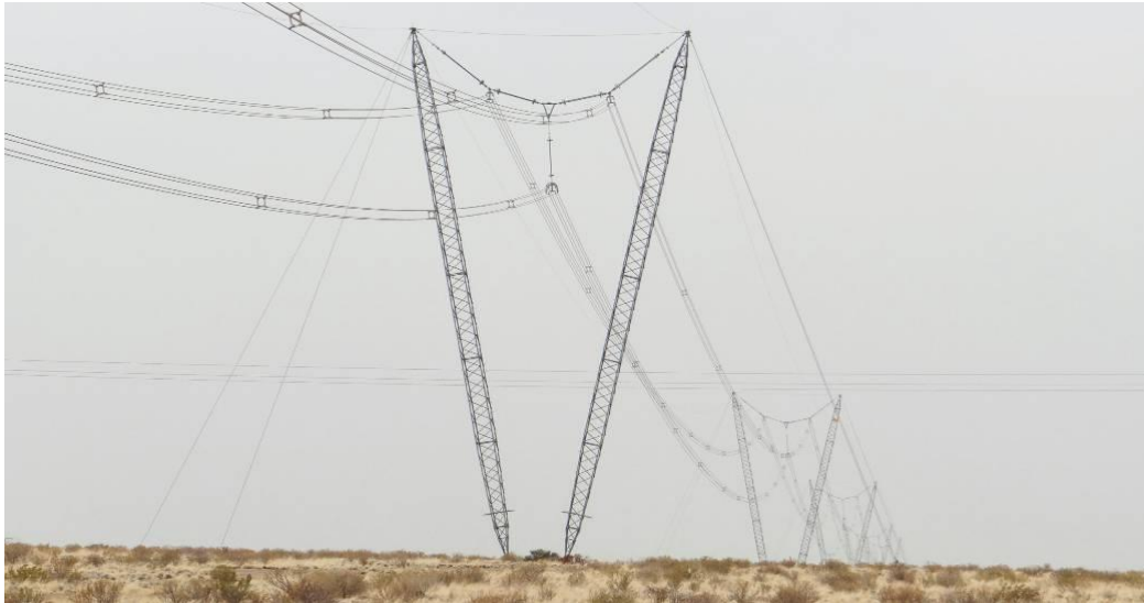
Photograph 1: A 400 kV transmission line with Guyed Compact Cross-Rope Suspension Towers. This illustrates what the proposed Kokerboom to Auas transmission line will look like in the straight sections of the alignment, where servitude constraints are not an issue.
