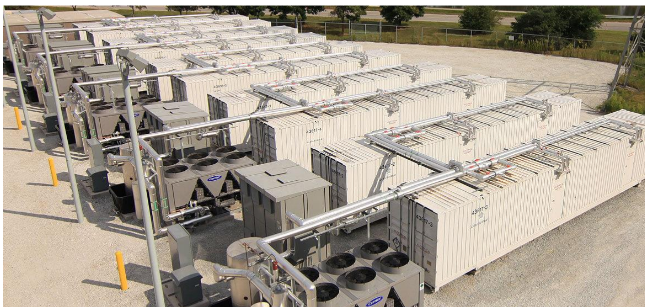
Figure 3: Typical containerized BESS facility (source: smart-energy.com)
