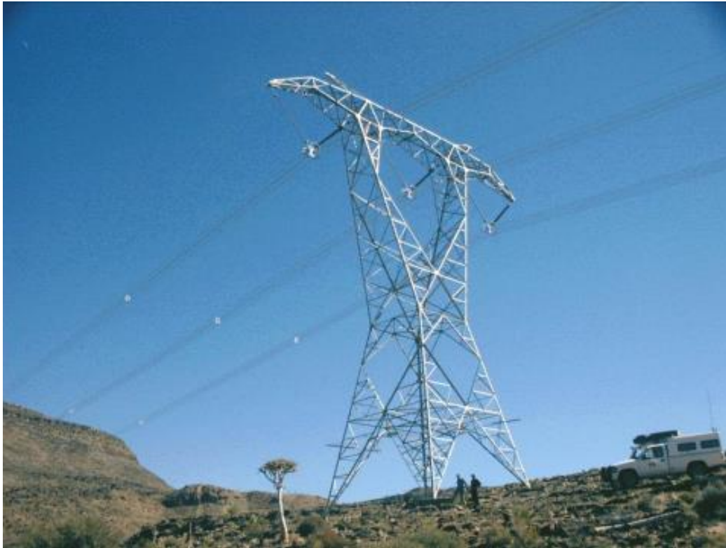
Photograph 3: Example of a Self-supporting Suspension Tower which would to be constructed within selected sections of the proposed Kokerboom to Auas transmission line, where the Guyed Compact Cross-Rope Suspension Tower would be impractical (eg at turning points and where there are servitude constraints).
