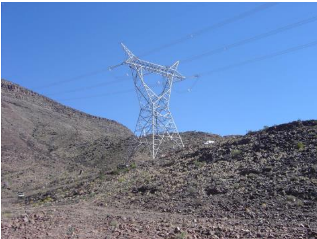
Photograph 1: A 400 kV transmission line with Guyed Compact Cross-Rope Suspension Towers. This illustrates what the proposed Kokerboom to Auas transmission line will look like in the straight sections of the alignment, where servitude constraints are not an issue.
